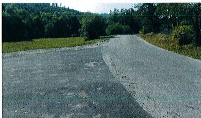
Km 63+957 (inceput drum, intersectie cu DJ136B)
